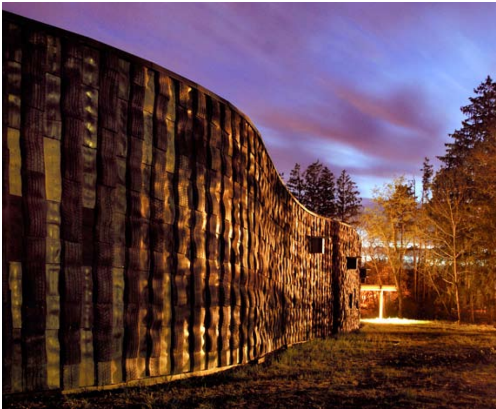
This photo, showing the north wall at dusk, highlights the tire shingles and entrance porch beyond.
