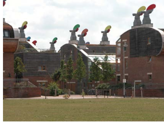
FIGURE 1. Beddington Zero Energy Development (2002). This project takes a holistic approach to energy reductions. It uses a combined heat and power plant to provide energy to the complex. Energy requirements are reduced through passive solar heating strategies. The project uses super insulation to assist with heat retention. Air conditioning is not provided. Wind cowls assist with natural ventilation for cooling. Designed by ZEDfactory.
