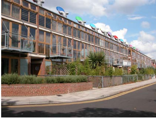
FIGURE 1. Beddington Zero Energy Development (2002). This project takes a holistic approach to energy reductions. It uses a combined heat and power plant to provide energy to the complex. Energy requirements are reduced through passive solar heating strategies. The project uses super insulation to assist with heat retention. Air conditioning is not provided. Wind cowls assist with natural ventilation for cooling. Designed by ZEDfactory.
