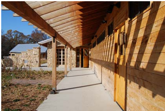
FIGURE 5. The Aldo Leopold Center started with the sustainable harvest of the Leopold forest. The wood was assessed and sized to maximize the number of structural columns and beams. The remaining wood whose diameter was insufficient was cut into smaller members as well as exterior and interior cladding. The structural system of the building was designed based on the materials list. This runs contrary to normal practices where the building is first designed and the materials ordered (even if limited to a close radius to reduce emissions impacts).
