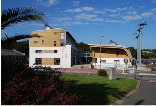
FIGURE 2. Jubilee Wharf, Penryn, UK (2006). This zero energy development uses 4 micro turbines to provide power. Evacuated tubes provide solar hot water. The roof has been designed for PV, but no PV is presently installed. Directional wind cowls assist with natural ventilation to the point that no A/C is provided. A 75kW wood pellet boiler provides under floor radiant heating. The building is super insulated with 300mm of insulation netting a U value of 0.1\text{W}/\text{m}^2/\text{k} . Designed by ZEDFactory.
