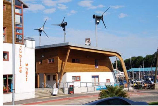
FIGURE 2. Jubilee Wharf, Penryn, UK (2006). This zero energy development uses 4 micro turbines to provide power. Evacuated tubes provide solar hot water. The roof has been designed for PV, but no PV is presently installed. Directional wind cowls assist with natural ventilation to the point that no A/C is provided. A 75kW wood pellet boiler provides under floor radiant heating. The building is super insulated with 300mm of insulation netting a U value of 0.1\text{W}/\text{m}^2/\text{k} . Designed by ZEDFactory.
