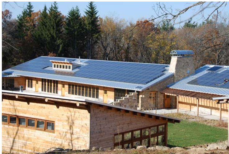
FIGURE 3. The Aldo Leopold Legacy Center, Bariboo, Wisconsin. This LEED™ Platinum building is also the first carbon neutral building in the United States. The conception of the design began with a budget and resultant area that would be dedicated to the installation of roof mounted photovoltaics. The building's energy use and size was designed with this limitation. Designed by Kubala Washatko Architects.
