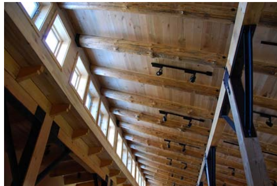
FIGURE 5. The Aldo Leopold Center started with the sustainable harvest of the Leopold forest. The wood was assessed and sized to maximize the number of structural columns and beams. The remaining wood whose diameter was insufficient was cut into smaller members as well as exterior and interior cladding. The structural system of the building was designed based on the materials list. This runs contrary to normal practices where the building is first designed and the materials ordered (even if limited to a close radius to reduce emissions impacts).
