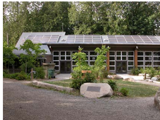
FIGURE 4. IslandWood, Bainbridge Island, Washington. The buildings for this LEED™ Gold Eco Retreat were all sited to maximize their solar potential. Construction was kept to 3% of the site to minimize disturbance and preserve the natural ecosystems on site. The roof of this education building is covered in PV to power the electrical needs of the classrooms. The building design uses passive principles and materials to retain heat and promote cooling. The roof is constructed in a butterfly shape to collect rainwater, which is directed for storage in a large cistern at the front left of the building. Although not specifically designed with carbon neutral as the focus, the project employs all of the base concepts that reduce demand and impact making zero carbon the next logical step. Designed by Mithun Architects.
