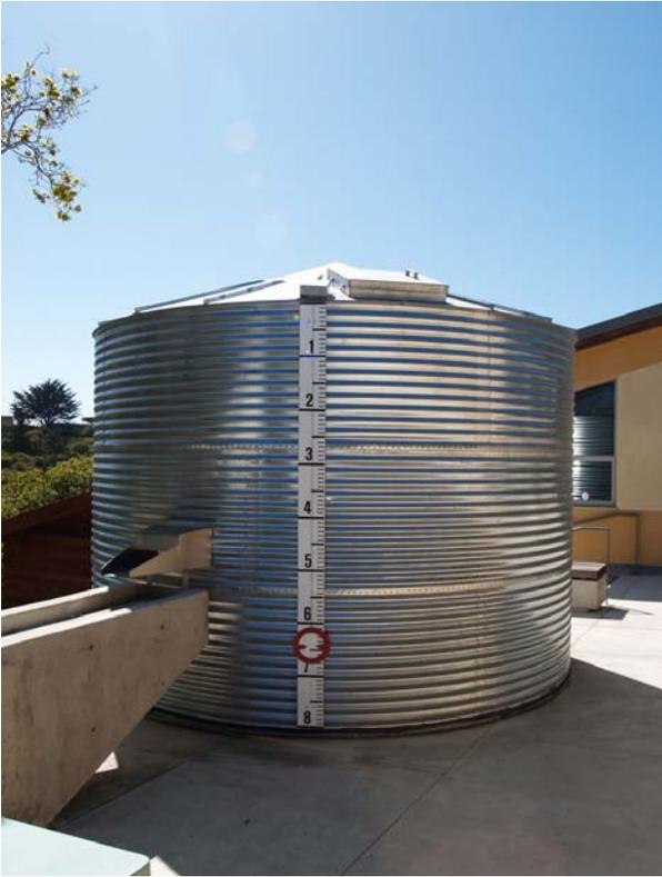
Fig. 11. Rainwater retention cistern with external display
