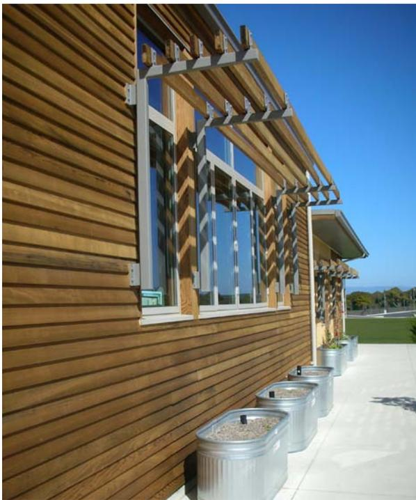
Fig. 9. Southern shading system and recycled wine-cask siding
