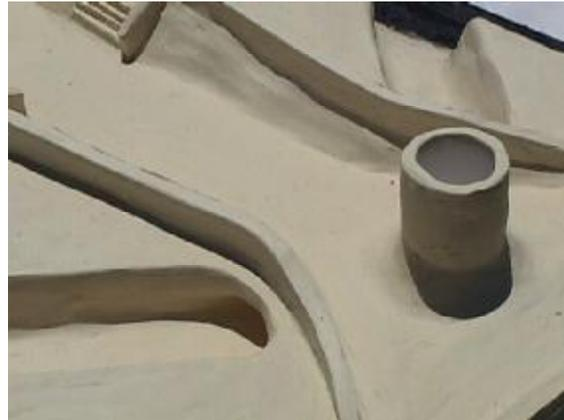
During construction, skaters are on the jobsite inspecting and adjusting the grading before rebar and shotcrete is placed, the last bit of “testing” the design receives before it is built. In our extensive use of shotcrete, we have seen it’s incredible flexibility to create non-linear designs and decided to use it together with grind rails to create a skateable building. The “cubistic rock” look fit nicely with the boulders found on this particular site.
