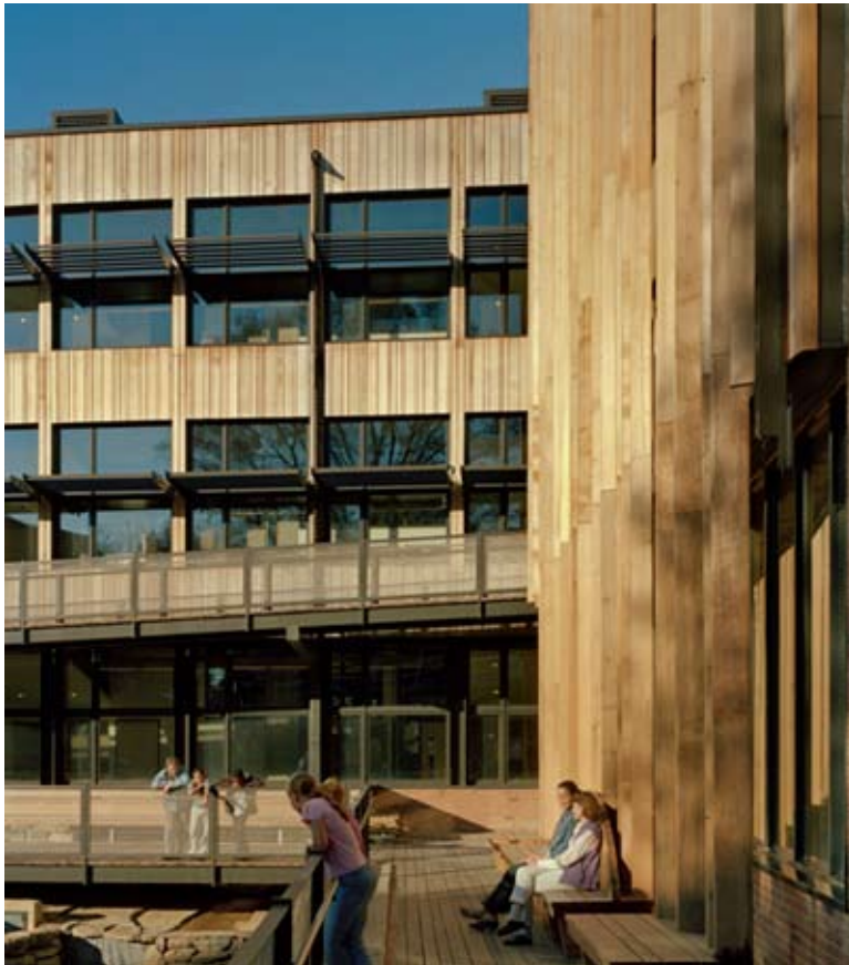
This photo highlights the exterior wood cladding.
