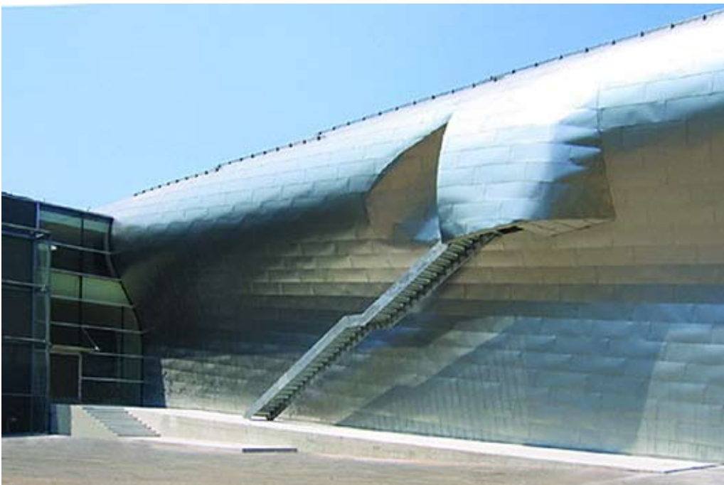
This photo highlights the building's stainless steel shingles.
