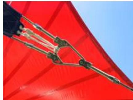
*Detail of stainless steel fittings, kevlar tie-back, and pvc fabric.*
