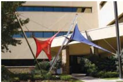
*One set of 'sails' was permanently installed at the main entrance to the UTSA College of Architecture. The realized project of tensile membrane structure closely resembles the design as envisioned by the class. (Image courtesy of the author.)*
