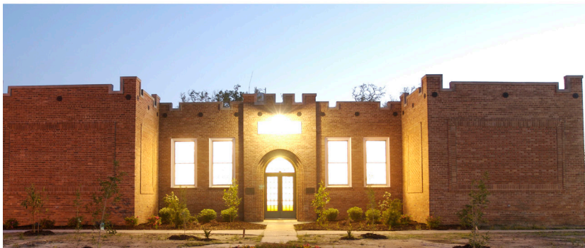
Old Waveland Elementary School post-Hurricane Katrina in 2005, and after restoration in 2008. Image credit: unabridged Architecture
