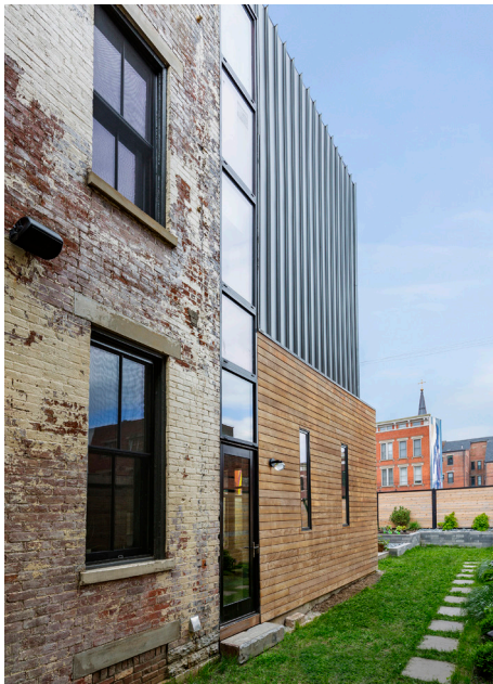
Myers-Heckman Side Exterior Image Credit: Sol design + consulting
