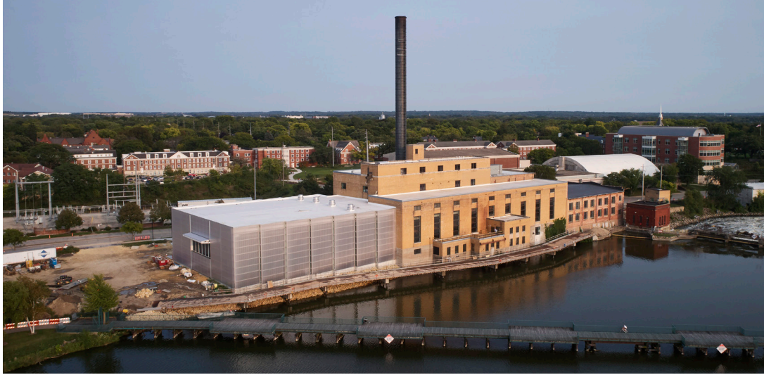
Beloit College Powerhouse Exterior | Image credit: © Tom Harris. Courtesy Studio Gang
