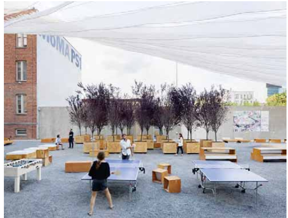
The temporary public space was shaded by a column-free, lightweight structure of ropes and retractable sails, that—strung from MoMA PS1's wall across the courtyard to the building's parapet—for the first time incorporated MoMA PS1's entire courtyard. Connecting the edges of the courtyard space, the structure revealed and reinforced the courtyard's very odd, idiosyncratic shape.
