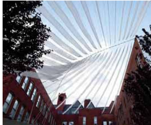
The temporary public space was shaded by a column-free, lightweight structure of ropes and retractable sails, that—strung from MoMA PS1's wall across the courtyard to the building's parapet—for the first time incorporated MoMA PS1's entire courtyard. Connecting the edges of the courtyard space, the structure revealed and reinforced the courtyard's very odd, idiosyncratic shape.
