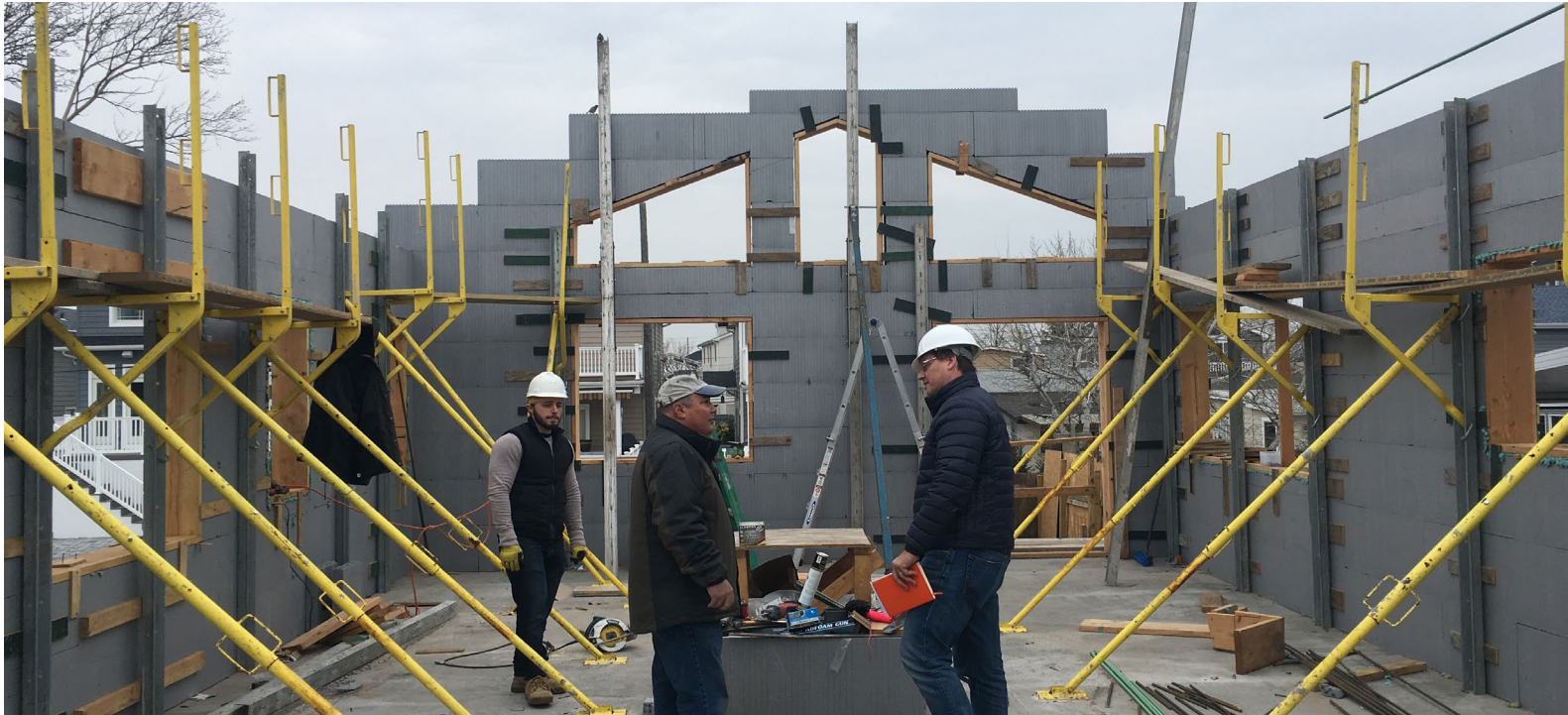
Hurricane Strong Home, ICF construction Image Credit: +lab Architect PLLC
