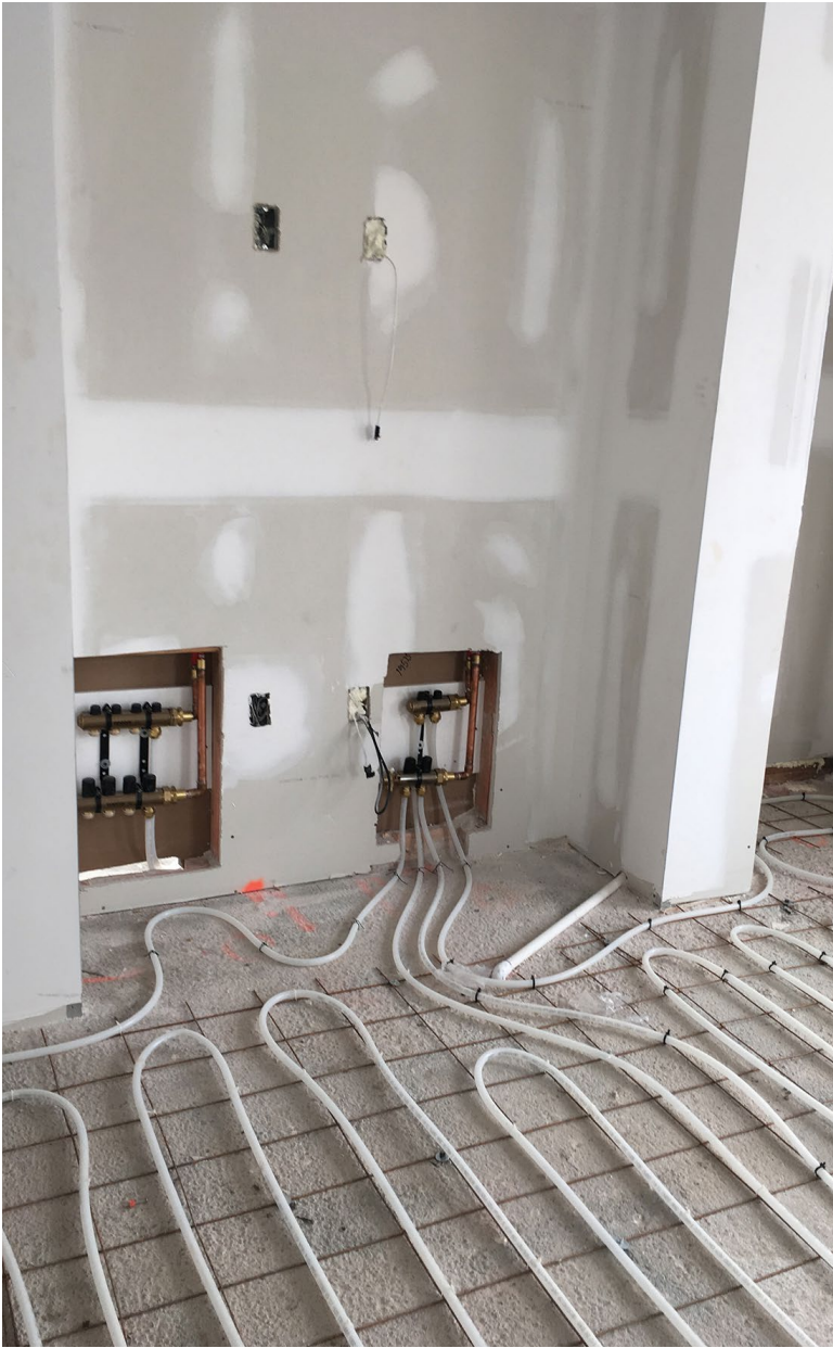
Hurricane Strong Home, Radiant floor heating installation in floor slab for thermal mass and comfort Image Credit: +lab Architect PLLC
