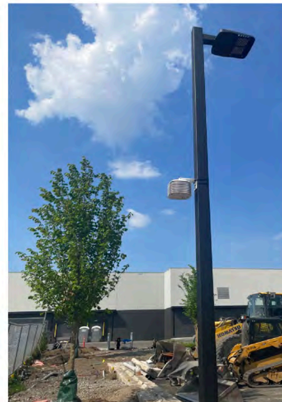
Sensors installed in both light poles and trees around the 22 Willow site.
