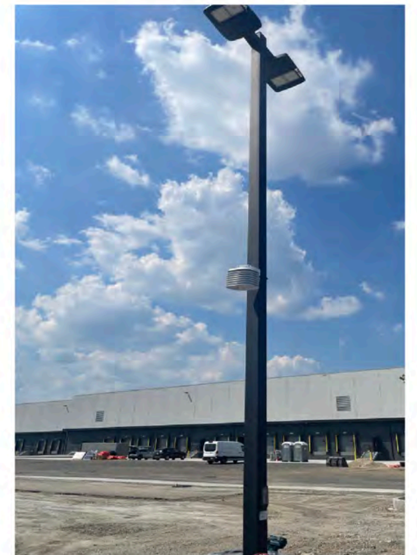
Sensors installed in both light poles and trees around the 22 Willow site.
