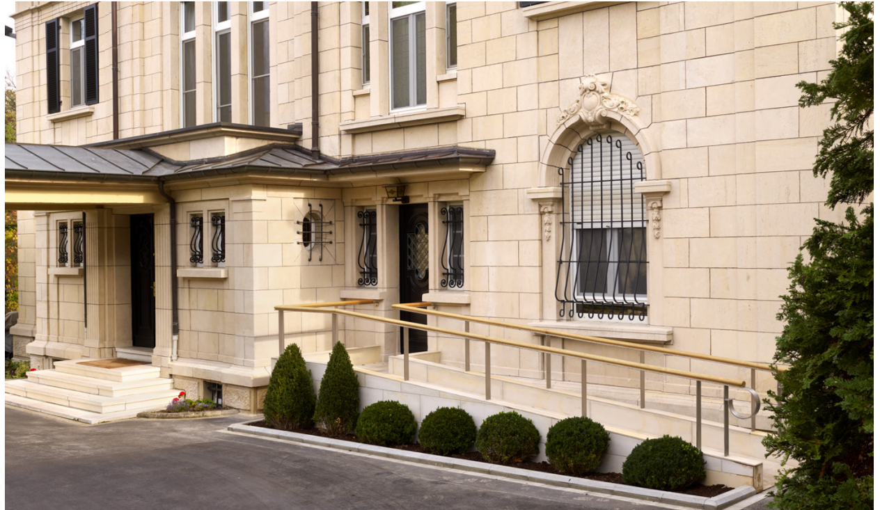
New accessible ramp at the Luxembourg Ambassador's residence provides access to diplomatic events for guests
