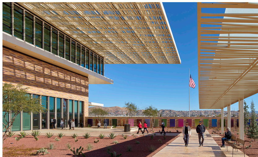
The ramada shade structure reduces heat gain on the façade reducing energy costs
