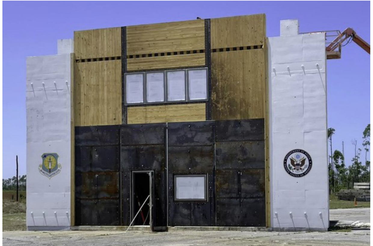
Mock-up of mass timber assembly for blast test
