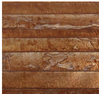
Custom, site formed weathering steel panels
