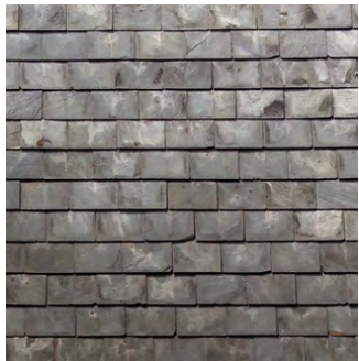
Discarded slate roof shingles repurposed as siding
