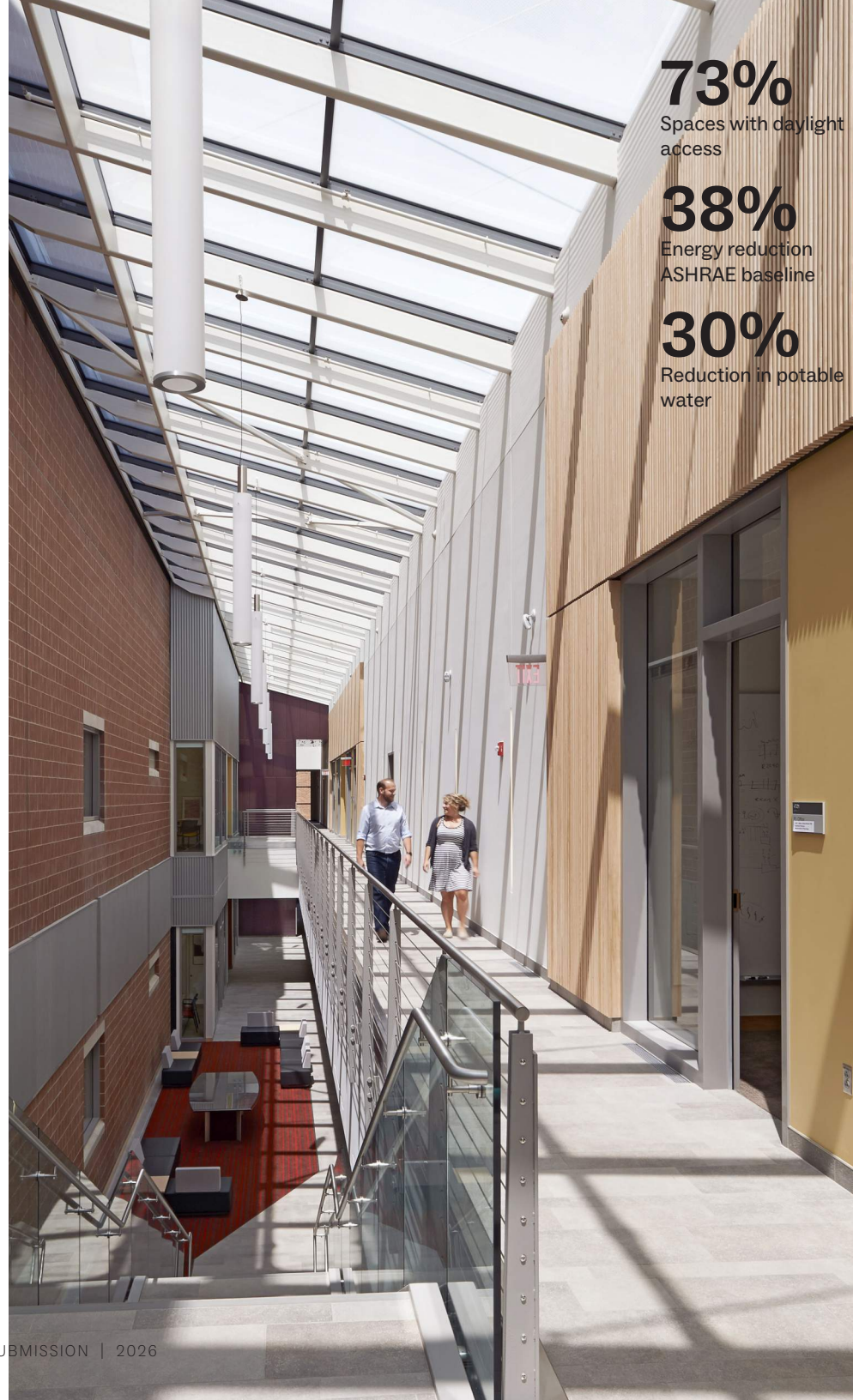
Daylighting analysis of the atrium meets IES targets (50 lux – circulation, 300 lux – work areas), with adopted recommendations including transom windows to improve daylighting in work areas and solar reflectors on existing walls to enhance sunlight penetration.
