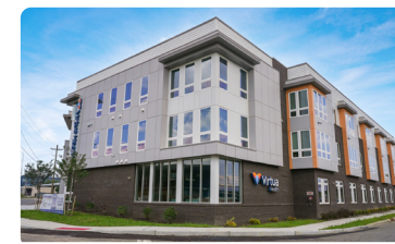
3.10 Built Work Creating Equitable Spaces Oliver Station and One Thompson Avenue
