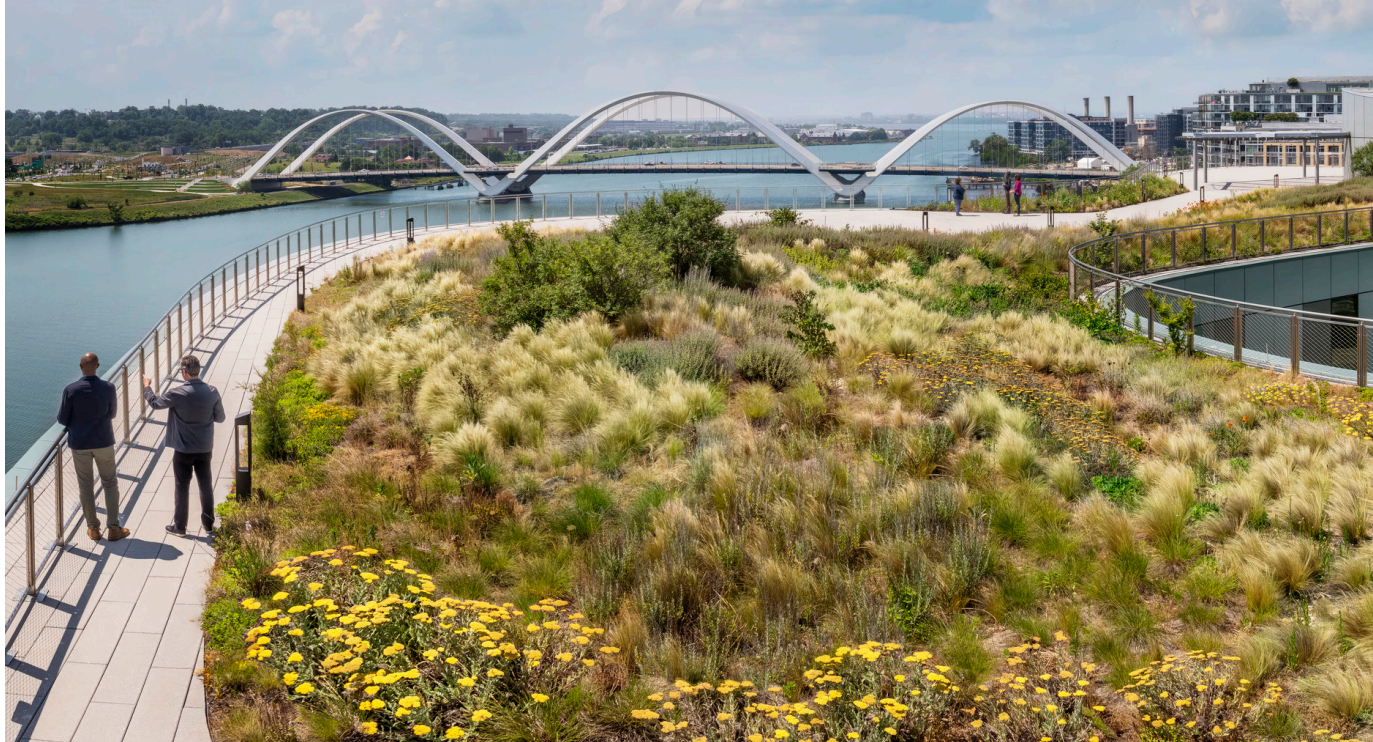
The stunning rooftop integrates a topographic green roof with hardscape, managing stormwater, while providing an amenity and event space.
