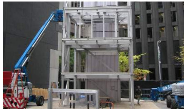
Kieran Timberlake, Cellophane house construction MoMA
