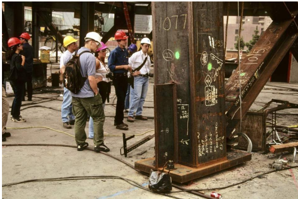
Frank Gehry - Disney Concert Hall construction site visit with Craig Webb
