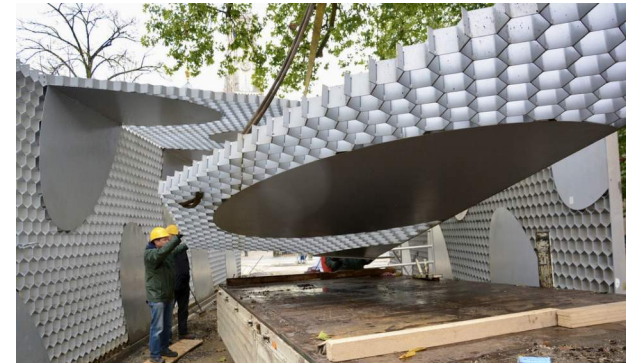
Toyo Ito - Brugge Pavilion Construction
