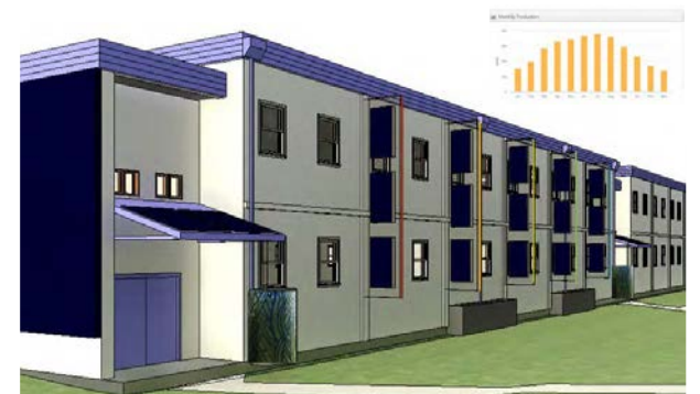
Building integrated photovoltaics (BIPV) on existing school
