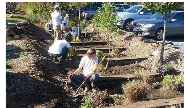
Monticello High School Biofilter Restoration, 2015
