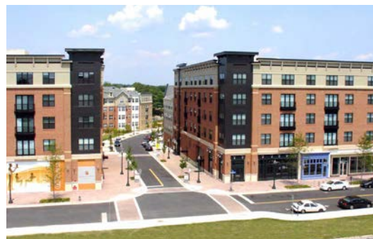
The Alaire at Twinbrook Station Rockville, MD, Role: Dir. Environmental Design, 2010, 330,000 sf, LEED-ND Gold
