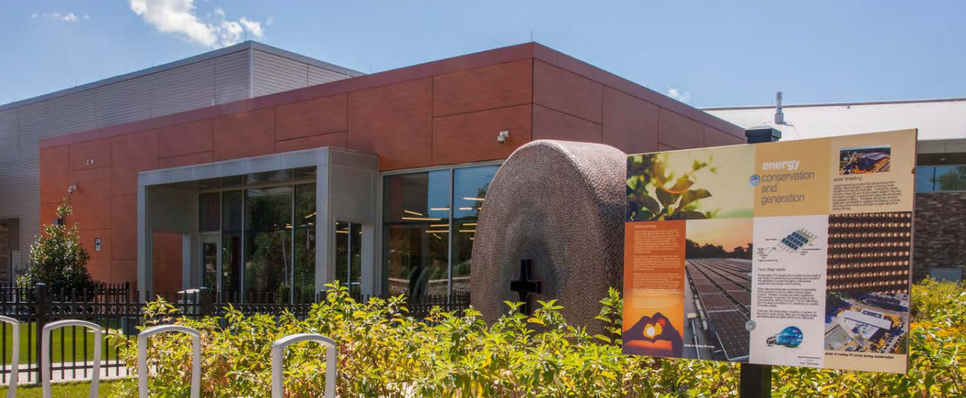
Educational signage in Emancipation Park explains Laurel Library's renewable energy system on the roof
