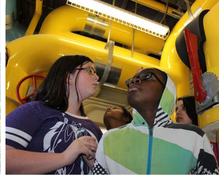
Student tour of the Geothermal Pump Room at Ducketts Lane
