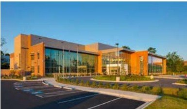
3.2 A NETWORK OF 25 SUSTAINABLE COMMUNITY BUILDINGS
