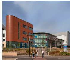
3.5 Walsall Manor Hospital, Walsall, UK: Unifying a Fragmented Campus
