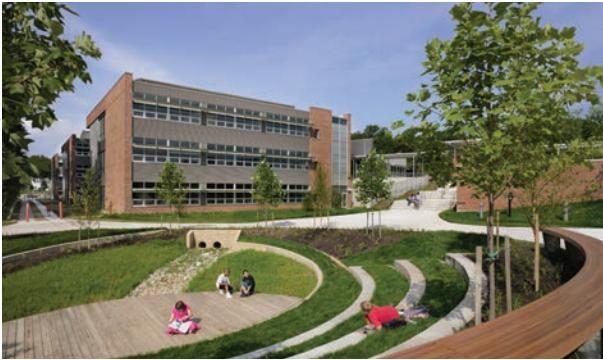
Manassas Park Elementary + Pre-K Manassas Park City Schools (Virginia) 2009 | Project Architect ( Exhibit 3.2 )
