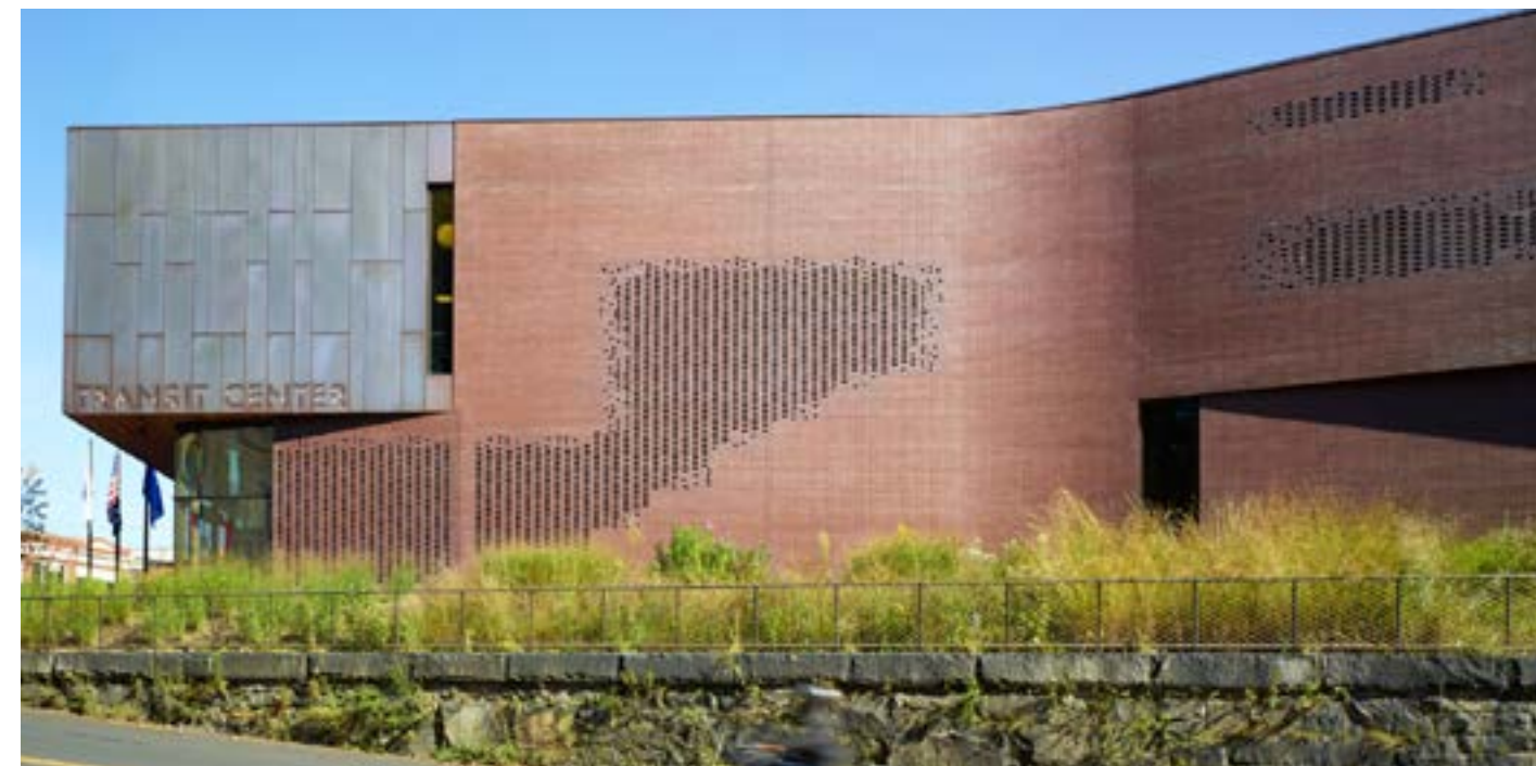
The John W. Olver Transit Center in Greenfield, Massachusetts balanced the programmatic needs of a transit center with the community needs for an county government office and with the natural need for native grassland. Image courtesy of Charles Rose Architects. Photo by John Linden.
