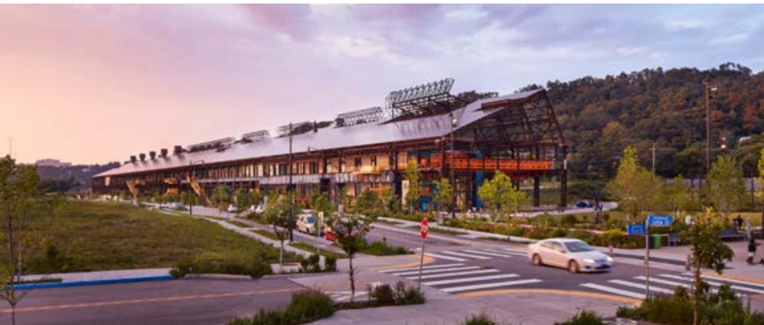
Mill 19 by RIDC and designed by MSR Architects and TEN x TEN as photographed by Corey Gaffer.
