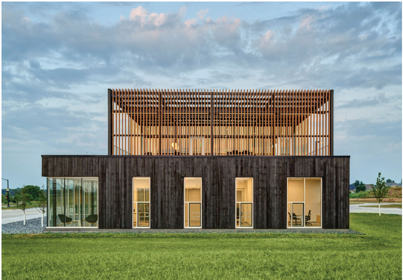
2026 COTE® Top Ten Award winner, Marion Fire Station No. 1, photo: Cameron Campbell/Integrated Studios
