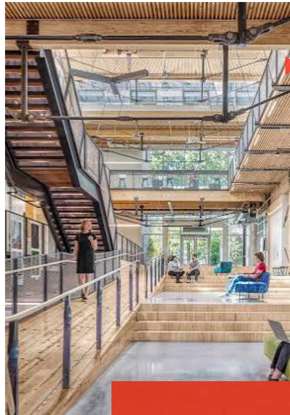
The Kendeda Building for Innovative Sustainable Design at Georgia Tech, Atlanta (The Miller Hull Partnership with Lord Aeck Sargent; Skanska, builder). The atrium ceiling is nail-laminated timber assembled from salvaged lumber, much of it from Atlanta's film industry, supplied through the Lifecycle Building Center. Photo: Jonathan Hillyer
