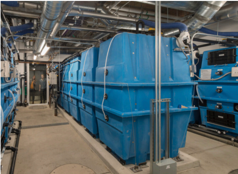
▶ The PAE Living Building in Portland, Oregon, utilizes a robust stormwater retention strategy, which captures and recycles rainwater three times. Photo credit: Lara Swimmer
