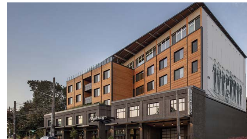
Seattle's Living Building Pilot Program helps incentivize projects like the Aegis Living Lake Union by Ankrom Moisan Architects. It is an assisted living and memory care community that achieved Living Building Challenge Petal Certification. Photo Credit: Magda Biernat Photography
