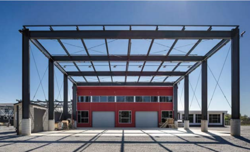
▶ The Construction Career Center under construction before the solar canopy was installed over “the yard” where students build large mock-ups and learn how to operate equipment. Photo credit: Holt Webb
